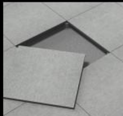
LAYING ON A RAISED FLOOR
